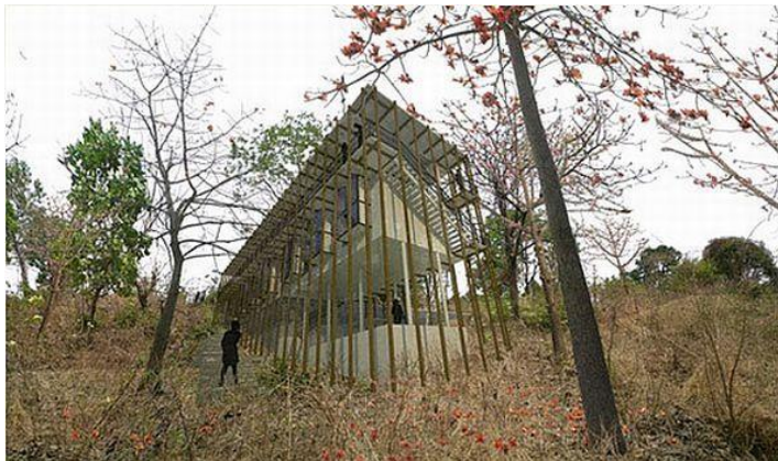
Figure 5: Multi storey building using Bamboo
